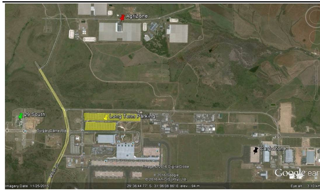
Figure 6.3 Photograph of solar panel installations for parking roofs
